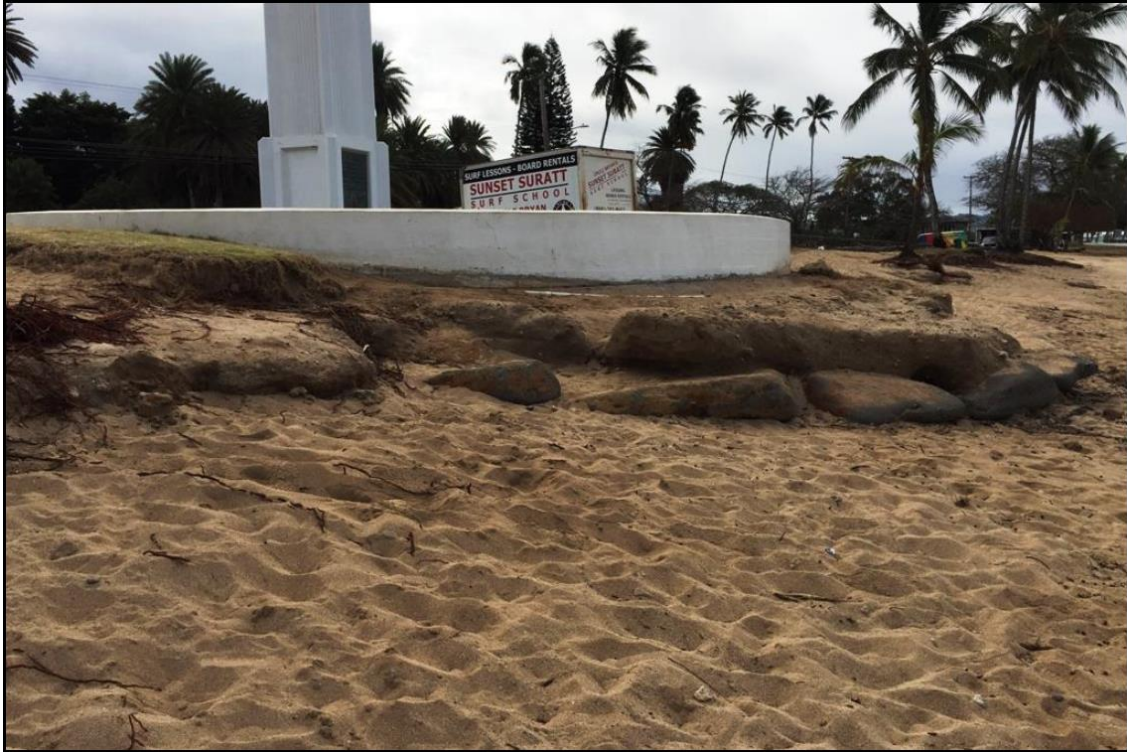
Figure 13. Erosion near WWII monument circa 2019 (SeaEngineering, 2019)
