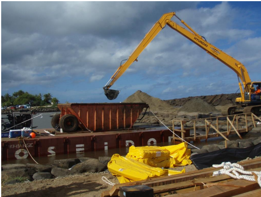
Figure A20. Typical method of mechanical dredging at Hale‘iwa Harbor (from 2009 construction)
