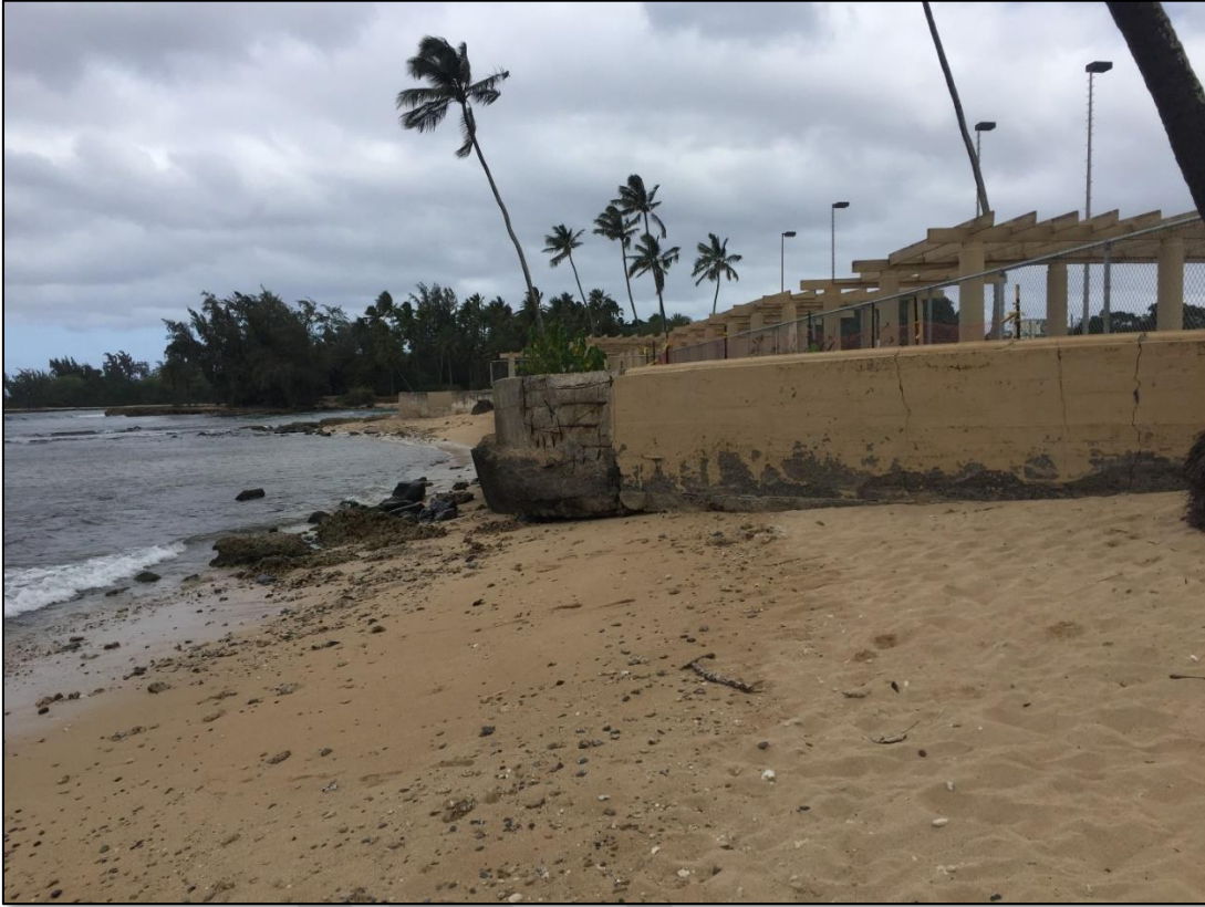
Figure 16: Hale'iwa Beach Park erosion.
