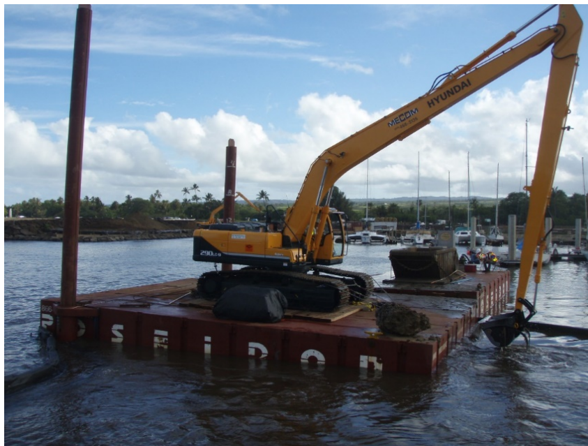
Figure 2. Photo of dredge operation during 2009 maintenance dredging.
