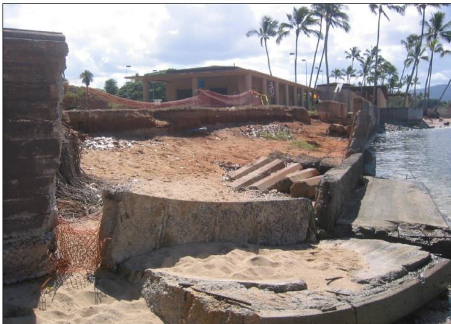
Figure 2-17 Damaged north end of wall (2008)
